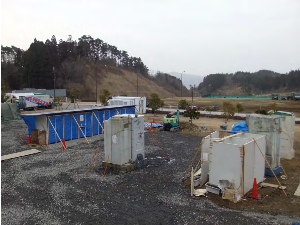
▲ The first task was the construction of makeshift toilets (foreground right). The construction took 2 days (toilets with blue sheets).
