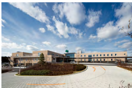
▲ Minamisanriku Hospital and Social Welfare Care Centre Minamisanriku
