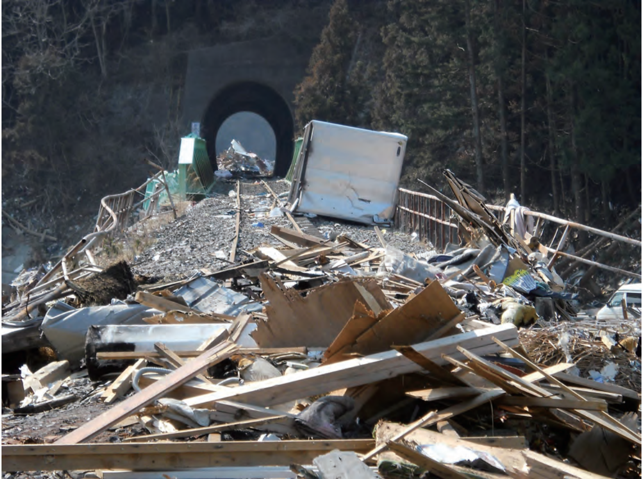
▲Elevated railroad tracks filled with debris.
